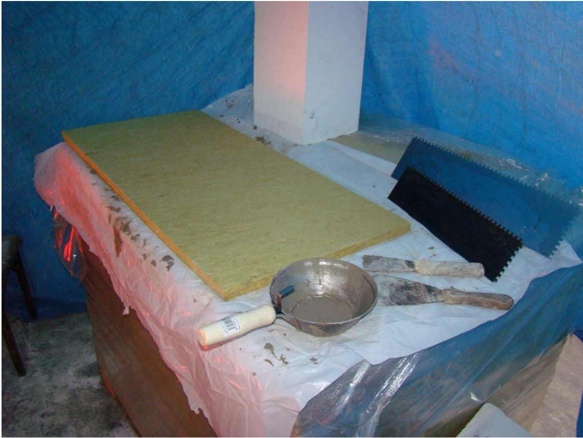
Inspect the slab and the tools used
