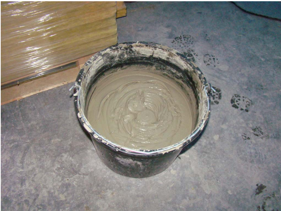
Prepare Dexaflamm B cement
