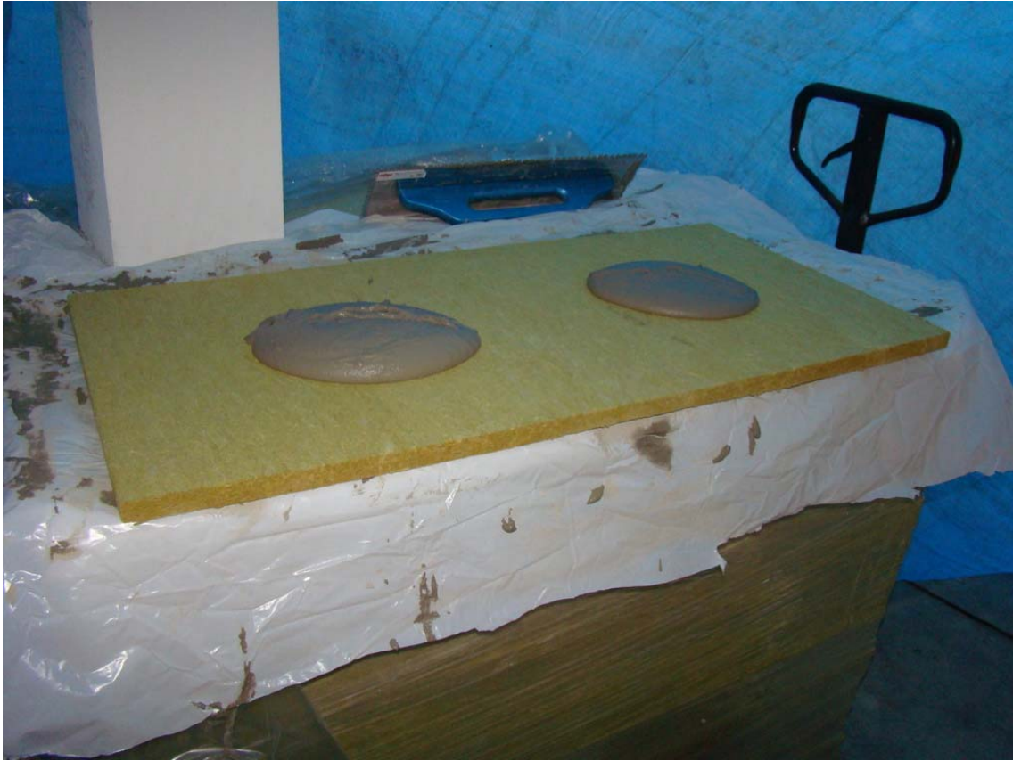
Apply an adequate amount of the cement on the slab
