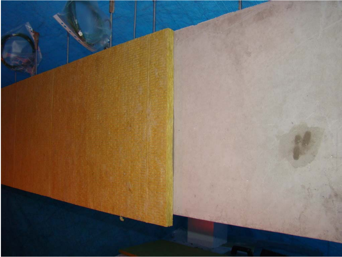
In case of a beam, the sides are glued first
