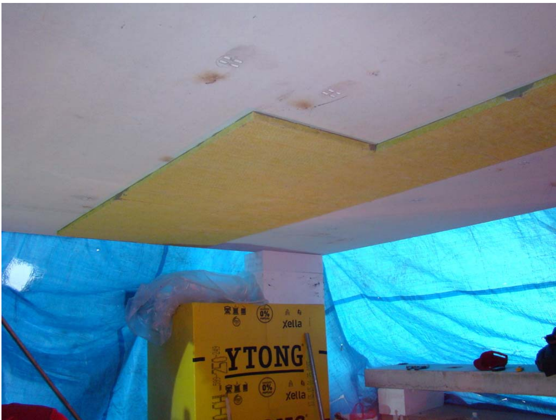
Install other slabs by pressing them against the edge of the already installed slabs (the edges are not glued)
